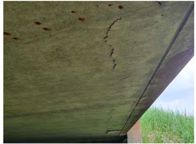
Looking at Delamination Along East Coping Full Length
