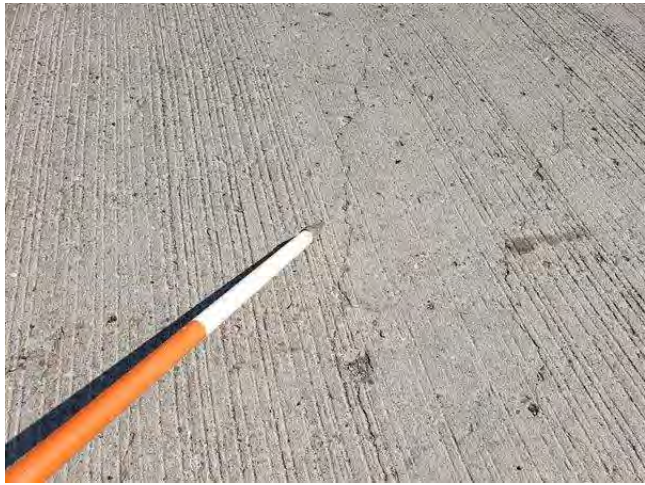
Looking at Deck Note-Transverse Cracks over Bent 3
