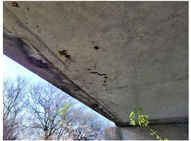
Looking at Spall and Delamination at East Face
