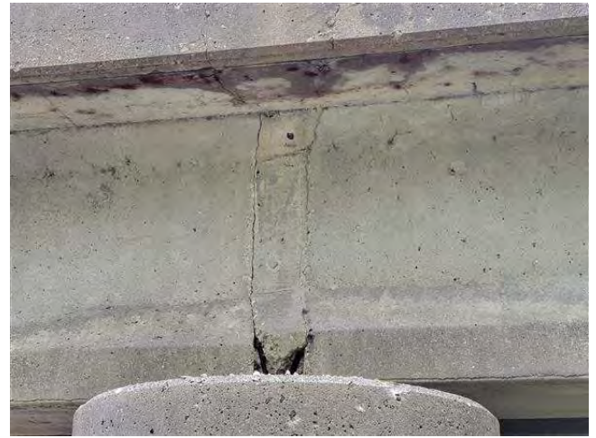
Looking at Spall at Beam Ends Pier 2 West Face
