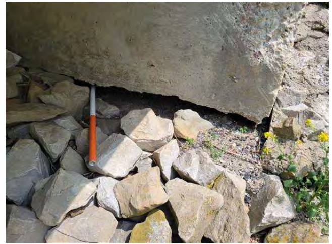
Looking at Undercutting at End Bent 4
