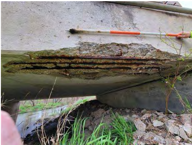
Looking at Large Spall With Exposed Reinforcement
