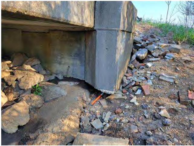
Looking at Undercutting of End Bent at Northeast Corner
