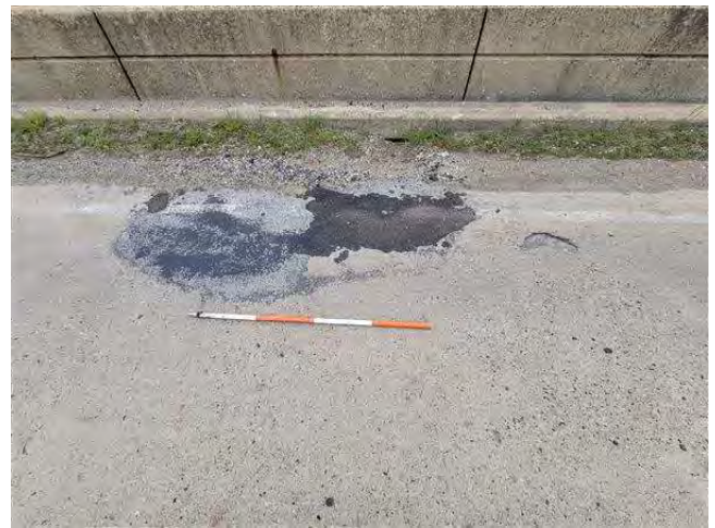
Looking at Asphalt Patch and Spall
