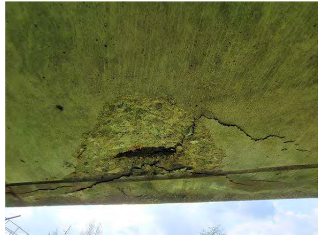
Lookign at Spall on Coping Span A
