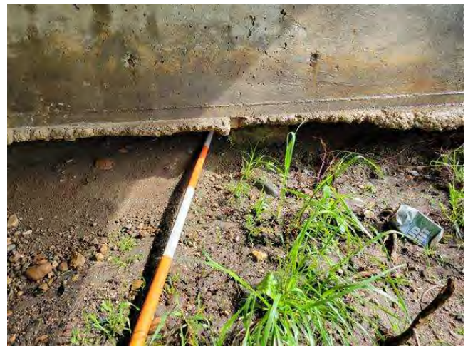
Looking at Undercutting at End Bent 4 with Exposed Pile
