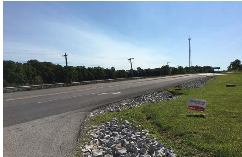
Existing road conditions include drainage swales and available right-of-way along SR32
