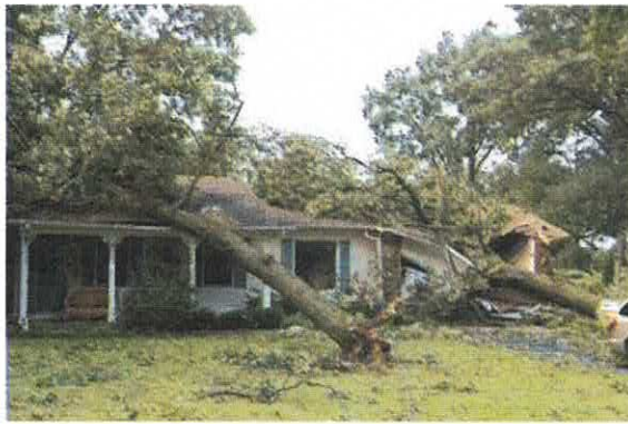
Figure 22 Home Damaged During Windstorm
