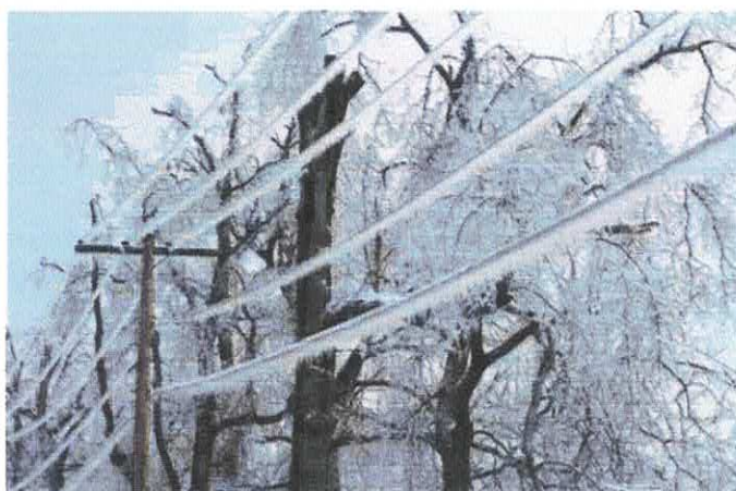
Figure 28 Ice Covered Power Lines
